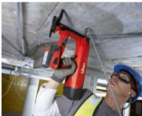
Threaded rod attachments to concrete
